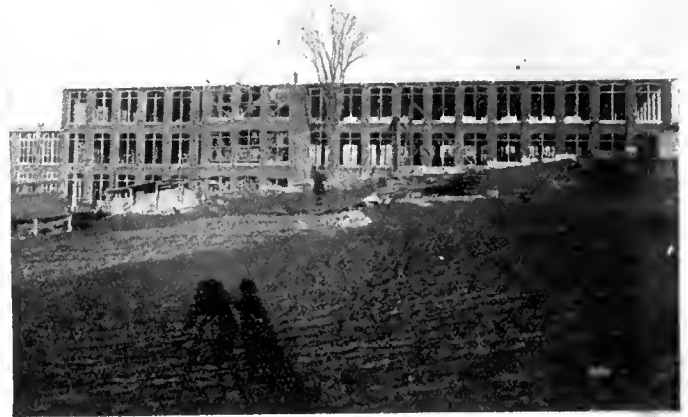
Fig. 4—New mill with roof completed.
